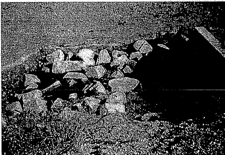
Figure 3. The use of loose rocks (riprap) to dissipate the energy of incoming runoff encourages mosquito production. Inevitably, standing water collects between the rocks, providing habitat for mosquitoes and making monitoring and control very difficult. A low-maintenance sloped concrete slab with imbedded rocks or concrete blocks is recommended as an alternative. Photo: Marco Metzger.
