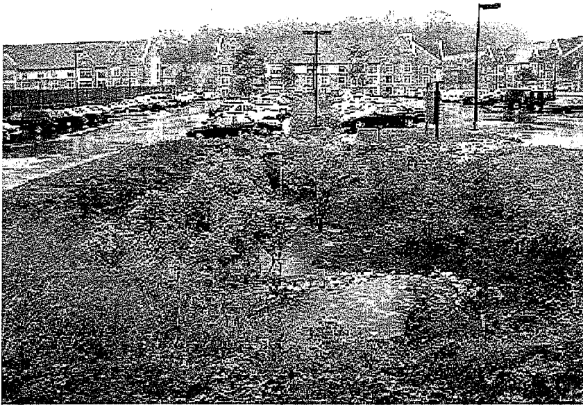
Figure 5-15. Biofilter Treating Runoff from a Parking Lot. Reprinted with permission from the Villanova Urban Stormwater Partnership (2005).
